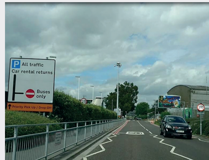
ADDITION OF GUARDRAIL APPROACHING THE AIRPORT
