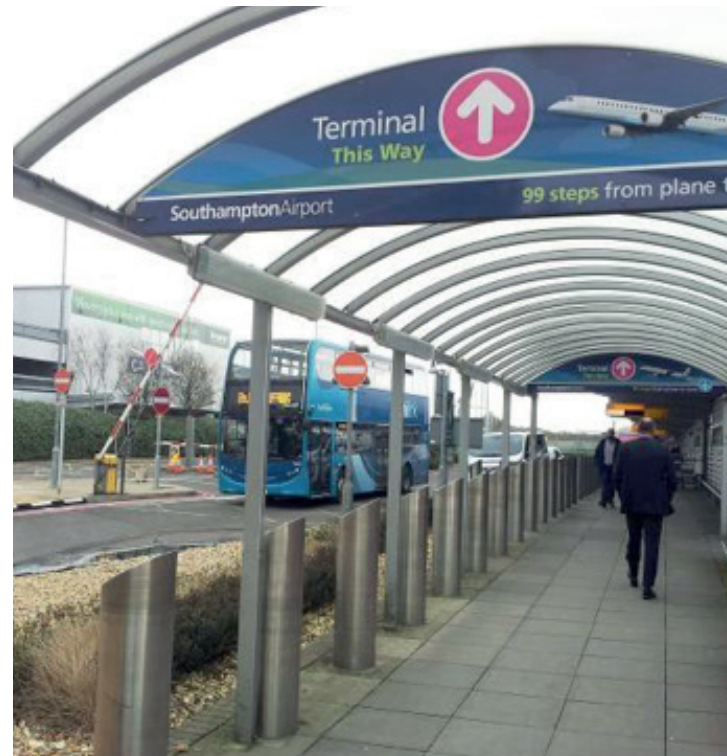
ENCLOSED PEDESTRIAN WALKWAY AND NEW PEDESTRIAN FOOTBRIDGE, WITH LIFTS PROVIDING IMPROVED ACCESS
