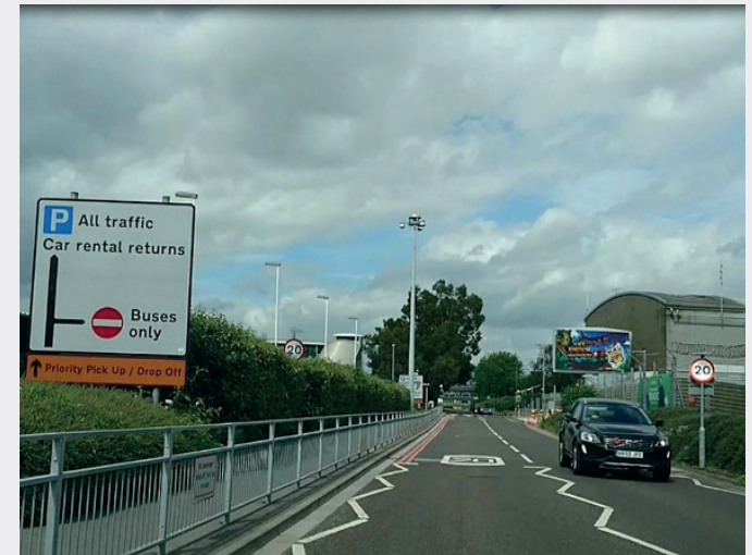
ADDITION OF GUARDRAIL APPROACHING THE AIRPORT
