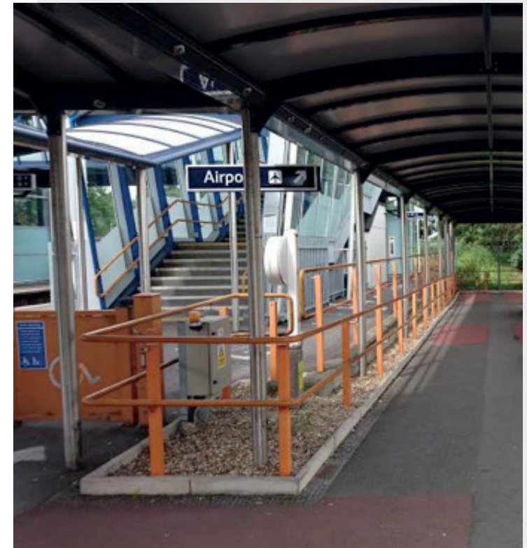
SOUTHAMPTON PARKWAY RAIL STATION
